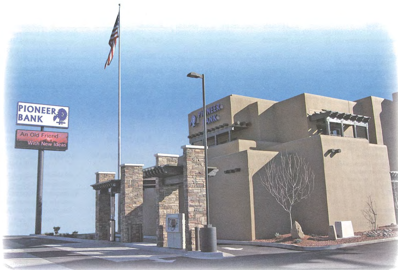
Pioneer Bank's Facility in El Paso - 6068 Gateway East
